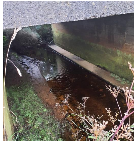
Photos of existing bridge
